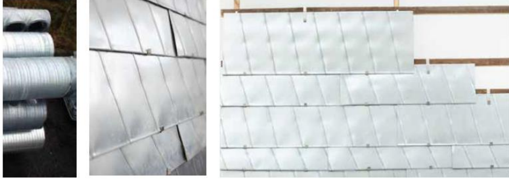
- Figure 39-41 / Details of the Spiro Facade system prototype. Left: sourced ventilation ducts.
