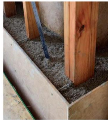
cast into formwork
