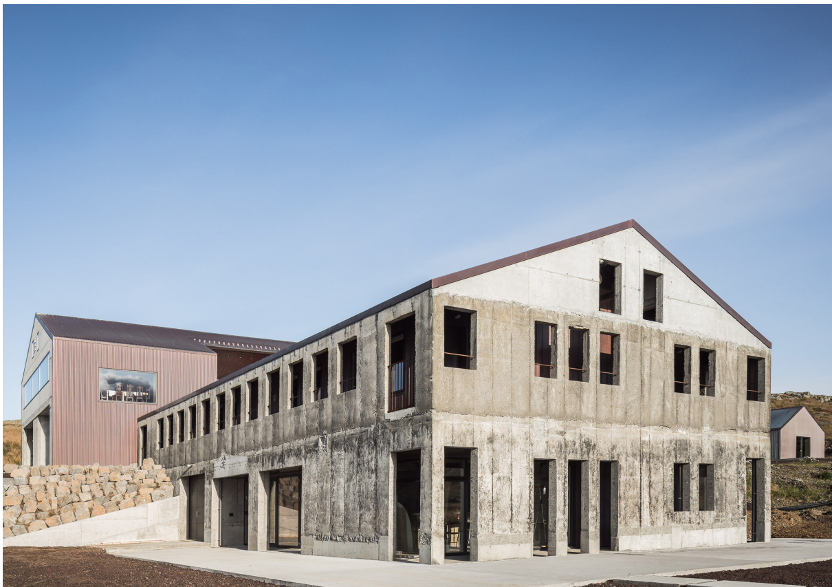
To maintain the original look of the cowshed, many of the new functions were placed inside the existing walls as independent structures © Estudio Gallardo
